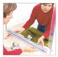
Be sure the edges and ends are in the correct position before contacting the mirror. Once on, the strip cannot be adjusted.
