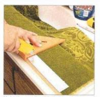
Hold the cutting blade low and keep it perpendicular to the surface so your cut goes straight into the acrylic.
