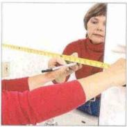
Two horizontal pieces are cut to a length that is 4 in. shorter than the horizontal measurement of the mirror.
