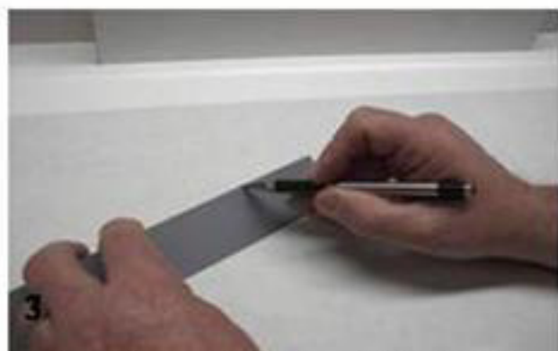
Transfer Center Marks to Rear of Mirr.Edge Strip
