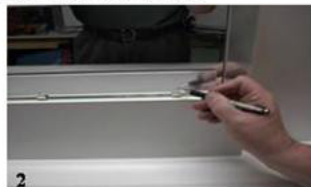
Install Vertical Mirr.Edge Strips. Place Horizontal Bottom Strip Above Clips and Mark Center Locations.
